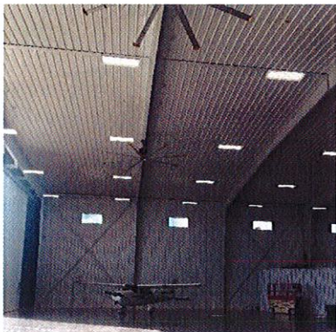
Interior Lighting – House of Raeford, Duplin County Airport
